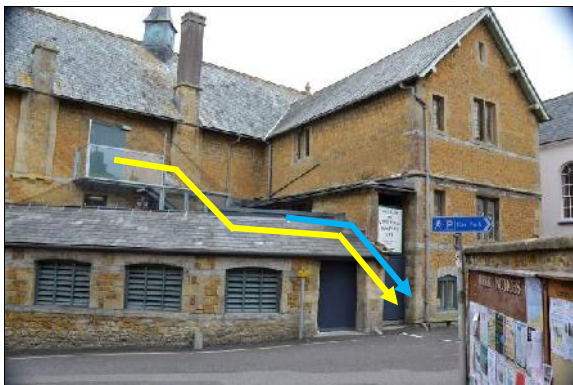
Images showing rear fire escape from 1 st and 2 nd floors
